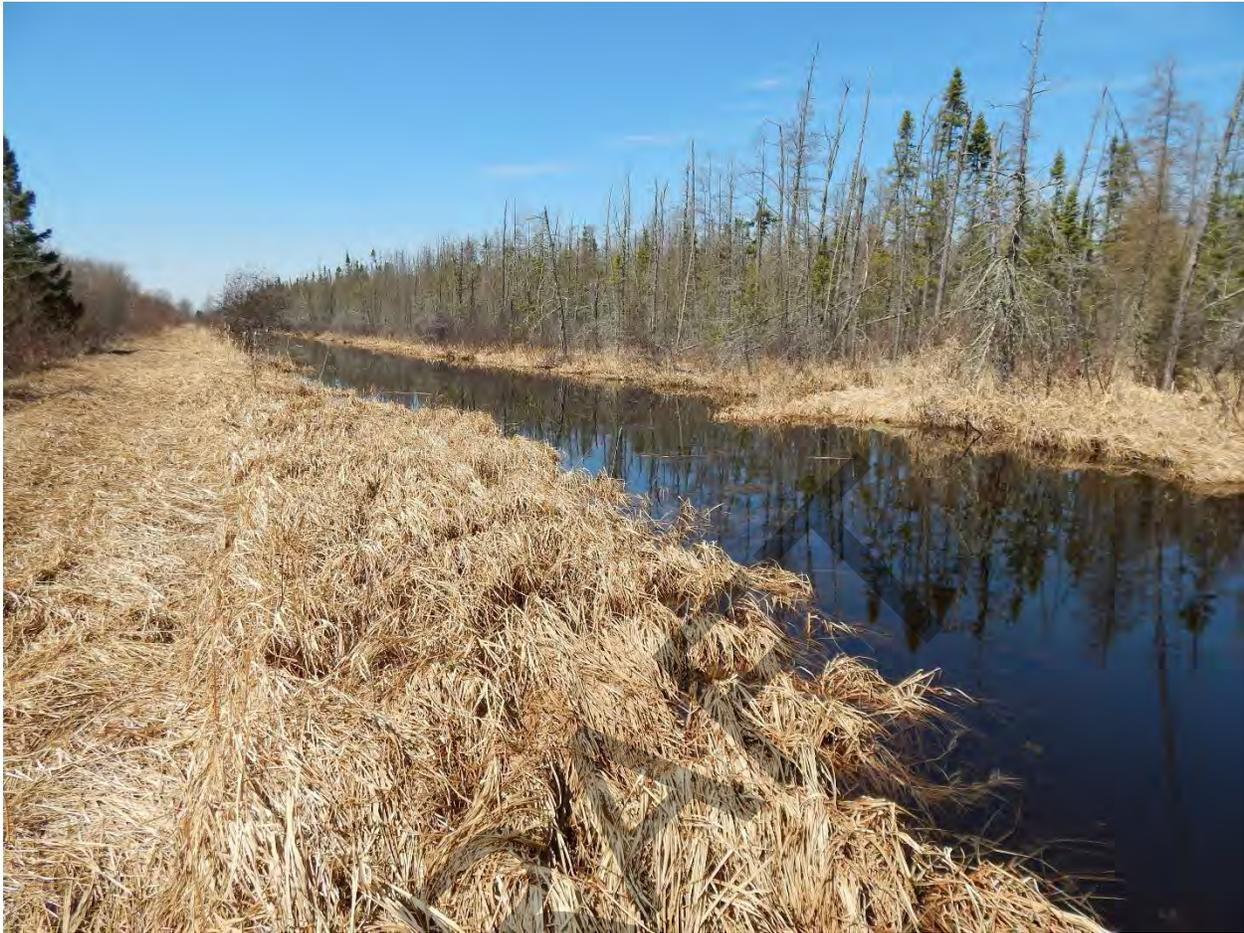
Image from same location shown in Graphic #6 and #7 with a westward aspect along the Lateral 7 Branch 1 corridor. Surface water elevation at the photo location was within 6” of overtopping the spoil at the date of the image. Evidence of weeping were encountered on the south side of the spoil, likely due to inconsistencies or decomposition of peat within the spoil alignment.
